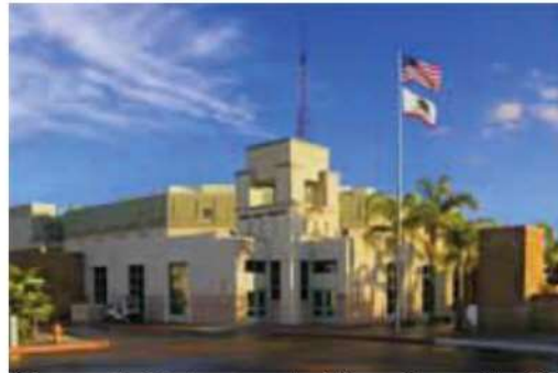
Figure 1. Entrance to Theo Lacy Facility Source: OCSD
