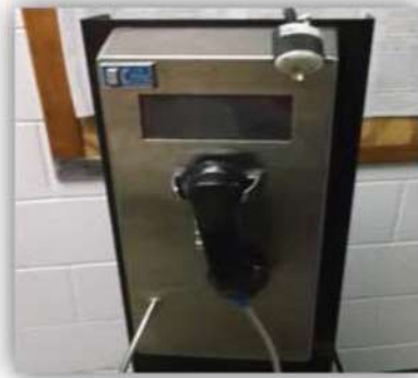
Figure 4. Broken plug on phone observed by OIG at TLF on November 16, 2016 Source: OIG
