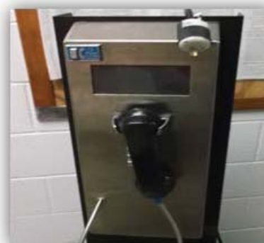
Figure 4. Broken plug on phone observed by OIG at TLF on November 16, 2016 Source: OIG
